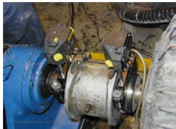
Figure 17. Setup of Laser Alignment Equipment
