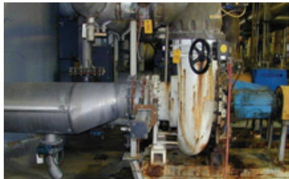
Figure 2. Eccentric Reducer on Suction Piping
