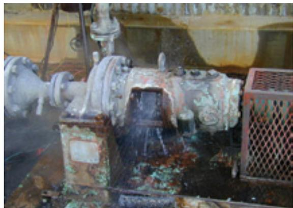
Figure 3. Concentric Reducer on Suction Piping
