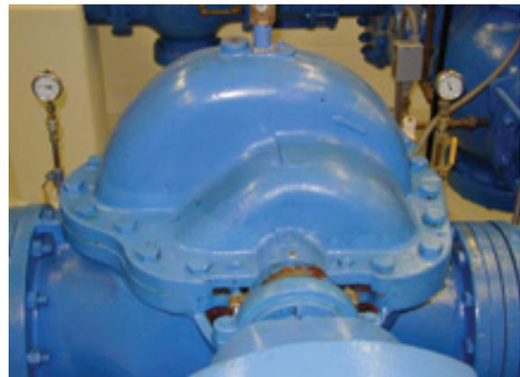
Figure 7. Double Suction Pump with Suction and Discharge Flange Pressure Measurement Connections
