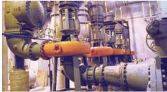
Figure 1. Eccentric Reducers on Suction Piping
